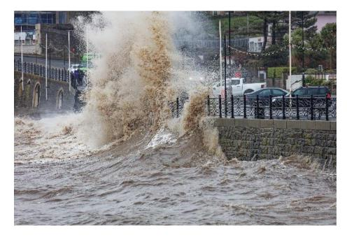
North Somerset has flood defences along the coast that provide a level of protection from storms. The defences are a mixture of walls, earth embankments and dunes. However, there is always a small risk that the storm will be larger than the defences have been designed for and could be overtopped, or a defence could fail.
